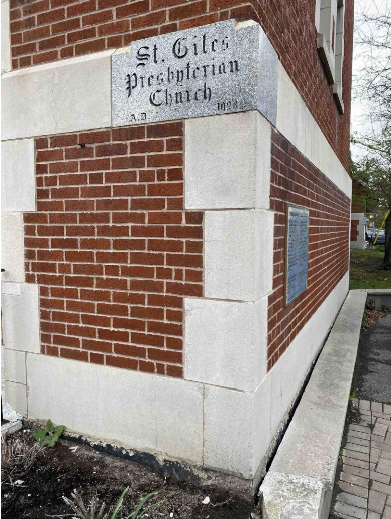
The Corner Stone of St. Giles Presbyterian Church (A.D. 1926), at the corner of Bank Street and First Avenue, Ottawa.
